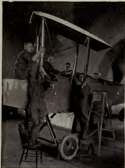
Figure 33—Assembly of center section
